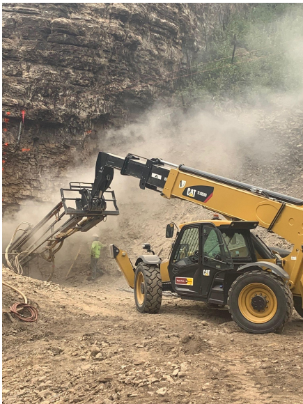
Drilling anchor for debris fence.
