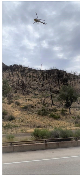
Xcel helicopter work last week.
